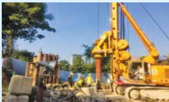
Piling works at the PNB118 Tunnel Project Site-1
