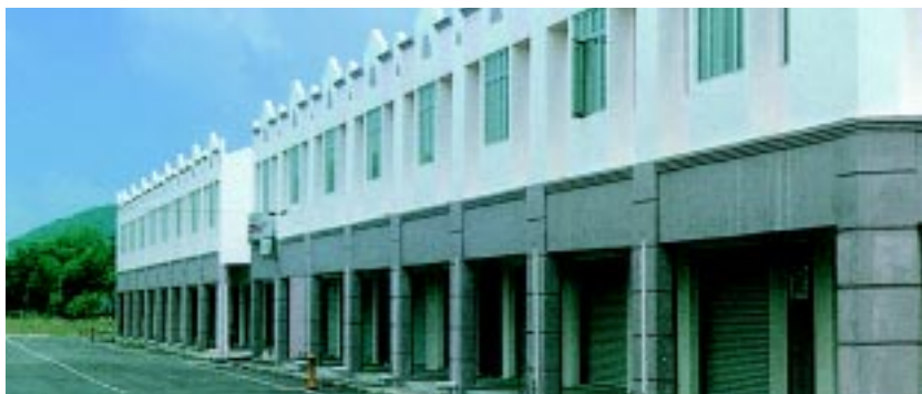
Completed Shoplots, Kerteh
