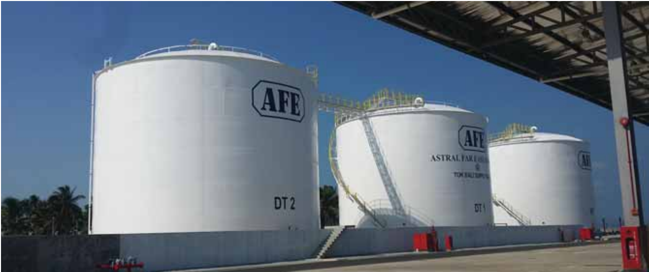
AFE Tank Farm at Tok Bali Supply Base.
