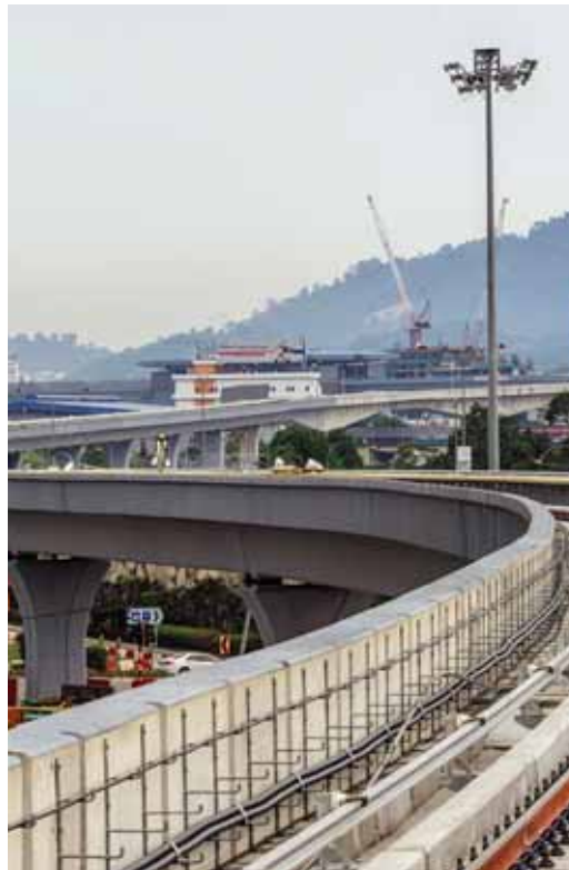
MRT Viaduct Guideway (package 6).
