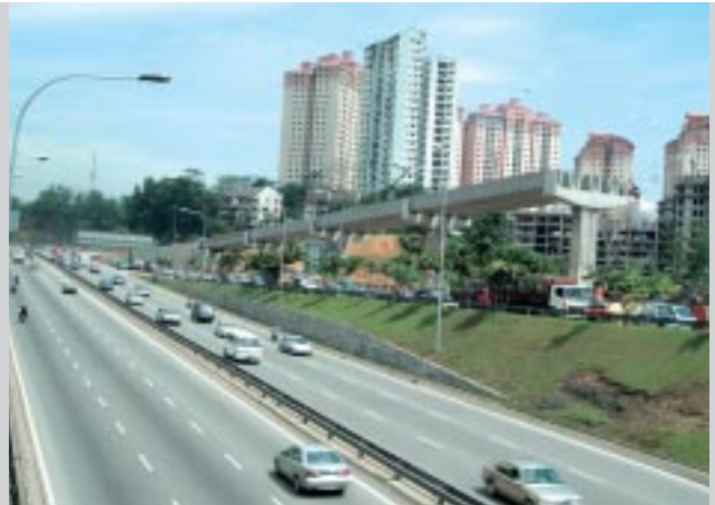
Construction work-in-progress at Jalan Duta
