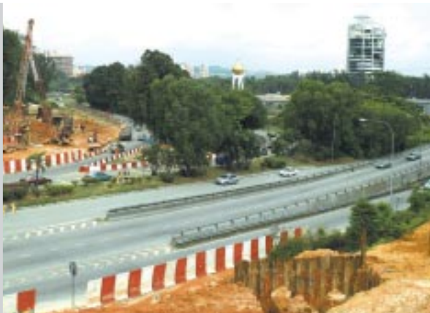
Construction work-in-progress at Jalan Subang
