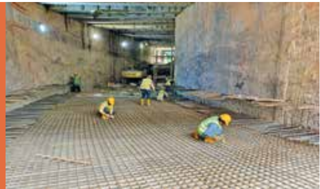
Installing rebar base slab VC sector at PNB118 Tunnels Project
