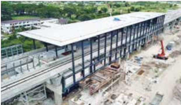
MRT Line 2 Package S206 - UPM Station in progress
