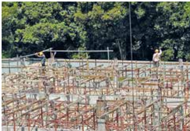
Railing work for roof beam area at POC Project
