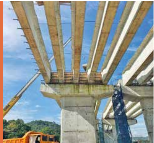
Concreting diaphragm in progress at EKVE
