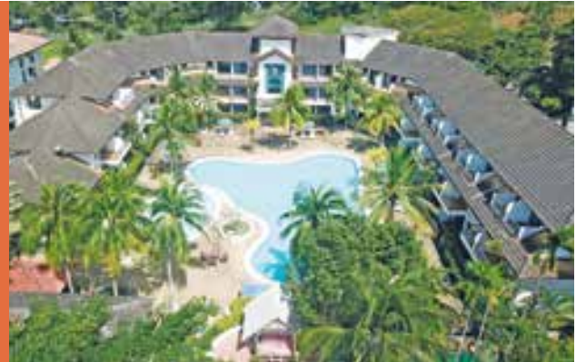
Residence Inn Cherating
